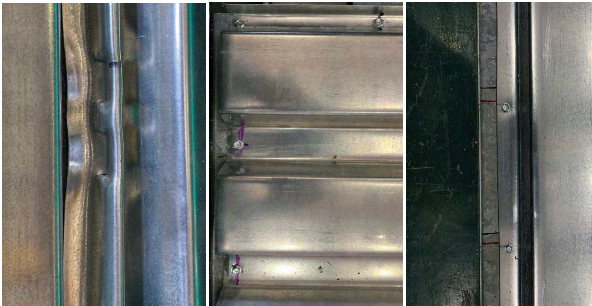
Figure 13: Typical sidelap (VSC-II), support (Hex-14), and edge connections (Hex-14)
